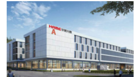
Energy Storage Manufacture Base
