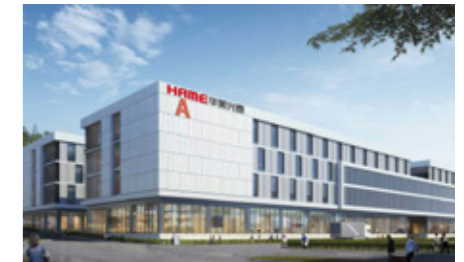
Energy Storage Manufacture Base
