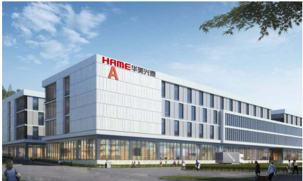
Energy Storage Manufacture Base
